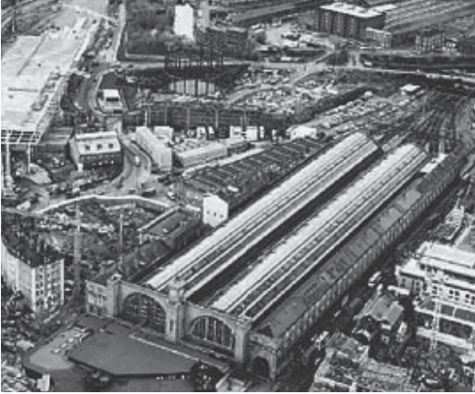
1 Kings Cross, London – urban redevelopment
